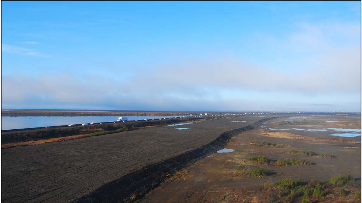
Setback levee built to protect SR 37 for the Cullinan Ranch tidal marsh restoration project, part of the USFWS San Pablo Bay National Wildlife Refuge. (Photo: Ducks Unlimited)
