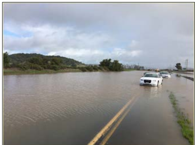
SR 37 flooding, January 23, 2017 (Photo: Sonoma County Transportation Authority)
