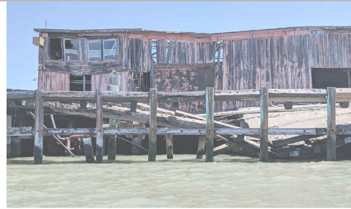
G G03/G04 EXISTING CONDITIONS - PHOTOS WAREHOUSE WHARF - WATER VIEW
