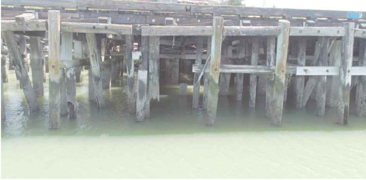
F G03/G04 EXISTING CONDITIONS - PHOTOS MAIN PIER - NORTH SIDE
