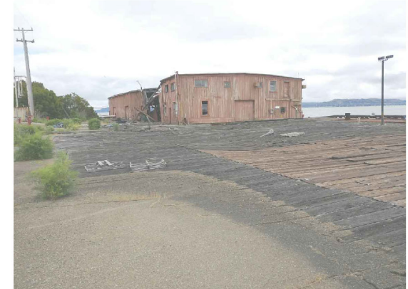
L G03/G04 EXISTING CONDITIONS - PHOTOS WAREHOUSE BUILDINGS - LAND VIEW
