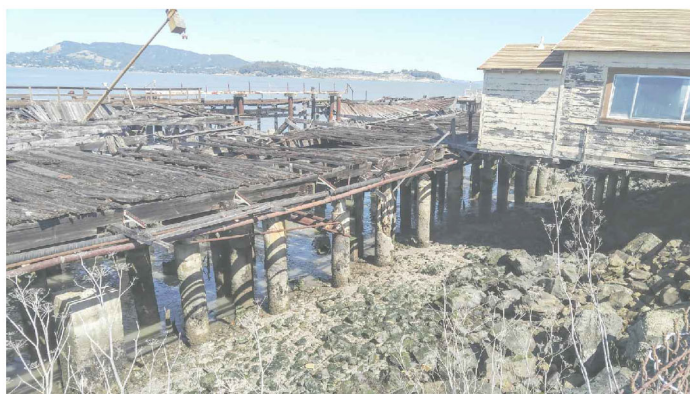
M G03/G04 EXISTING CONDITIONS - PHOTOS NORTH PILES - LAND VIEW
