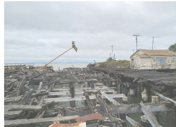
O G03/G04 EXISTING CONDITIONS - PHOTOS NORTH PILES AND OFFICE BUILDING
