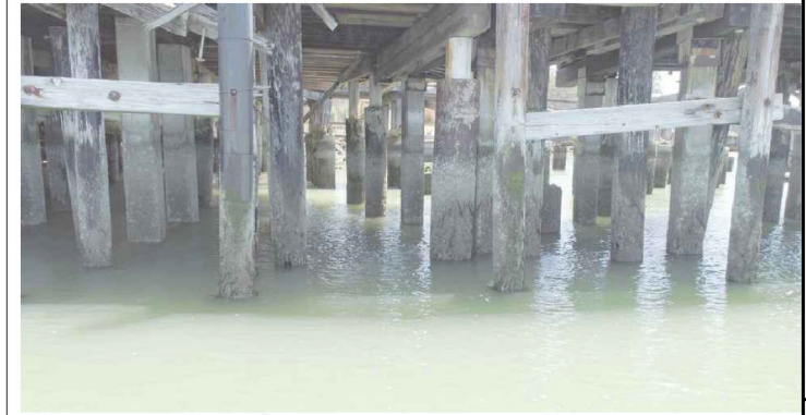
H G03/G04 EXISTING CONDITIONS - PHOTOS MAIN PIER - SOUTH SIDE
