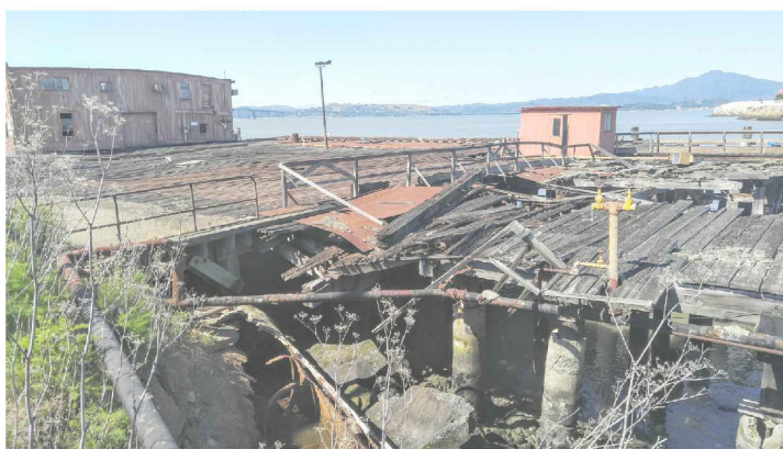
N G03/G04 EXISTING CONDITIONS - PHOTOS NORTH DECK - LAND VIEW
