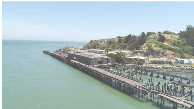
I G03/G04 EXISTING CONDITIONS - PHOTOS AERIAL SOUTH, WATER VIEW
