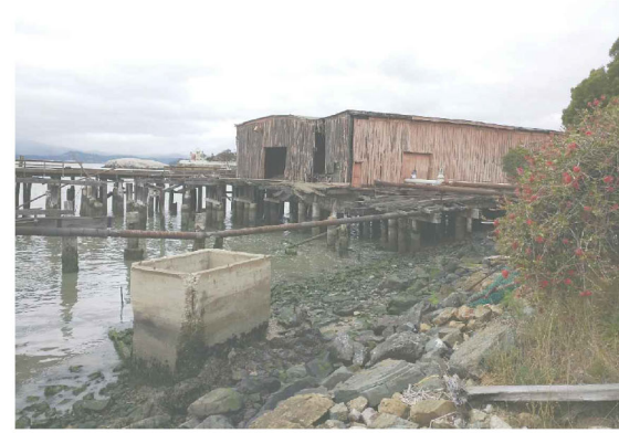
J G03/G04 EXISTING CONDITIONS - PHOTOS SOUTHEAST - LAND VIEW
