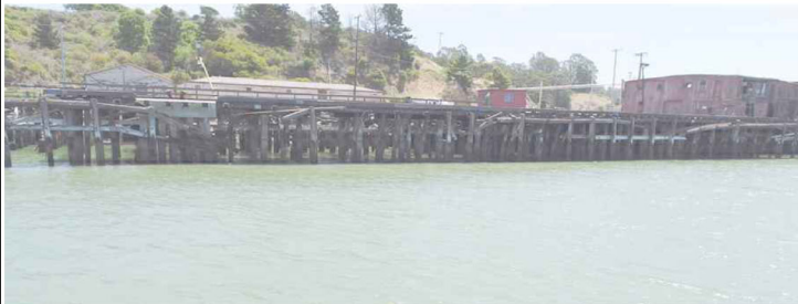
E G03/G04 EXISTING CONDITIONS - PHOTOS NORTH END - WATER VIEW
