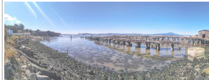
K G03/G04 EXISTING CONDITIONS - PHOTOS SOUTH PILES - LAND VIEW
