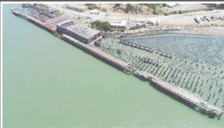
A G03/G04 EXISTING CONDITIONS - PHOTOS AERIAL OVERALL
