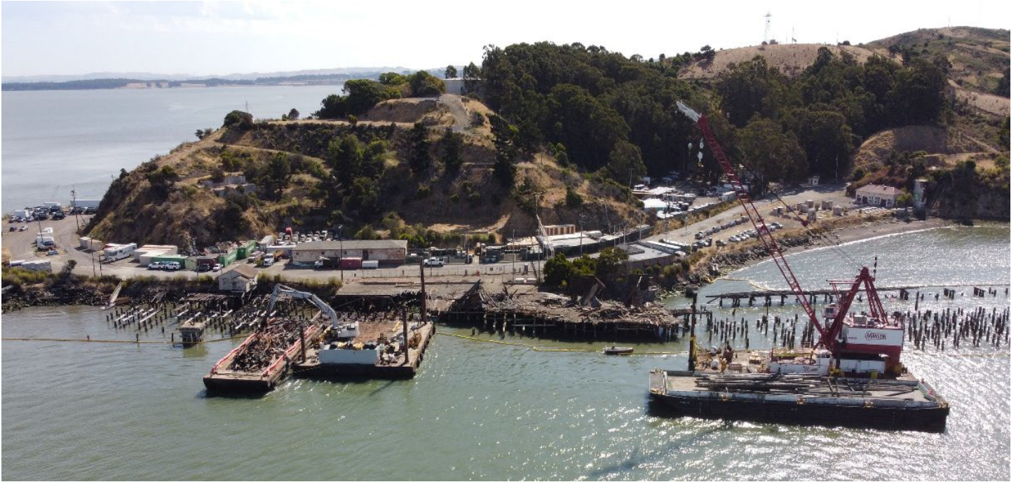
Wharf removal at Terminal 4 in Richmond
