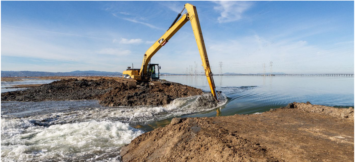
Breach of the Ravenswood R4 Pond, part of the South Bay Salt Pond Restoration Project
