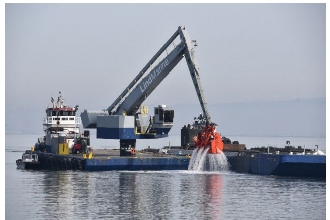
Dredged sediment being strategically placed in the SF Bay. Photo: USACE
