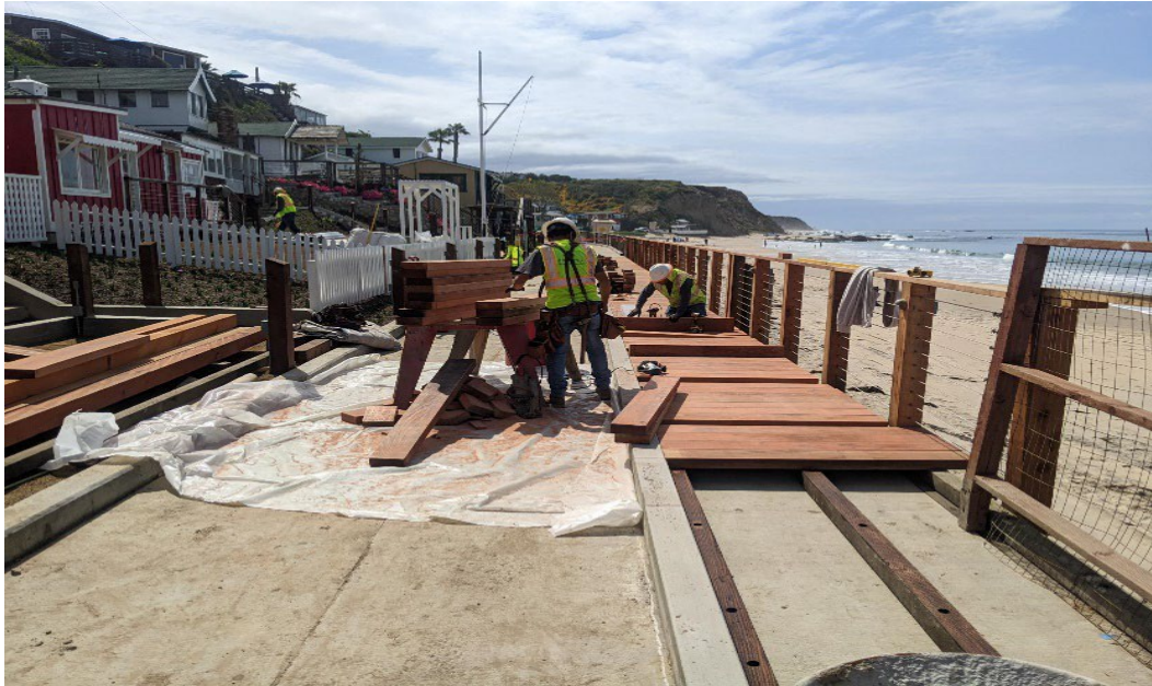
Construction at Crystal Cove
