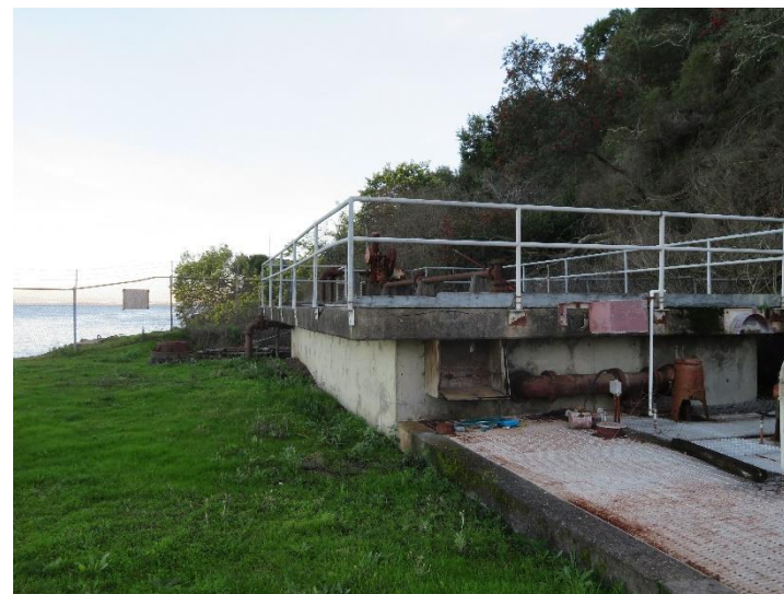
Defunct Water Treatment Plant
