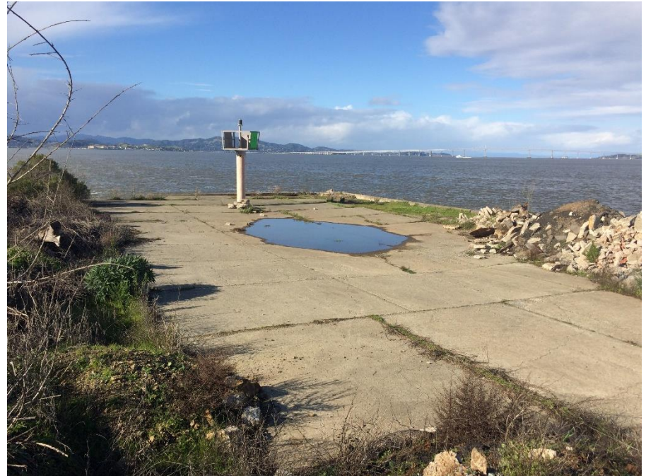
Backfilled area behind seawall, looking NE
