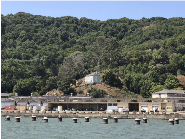
Existing Seawall, Slab and University Buildings in Central Reach
