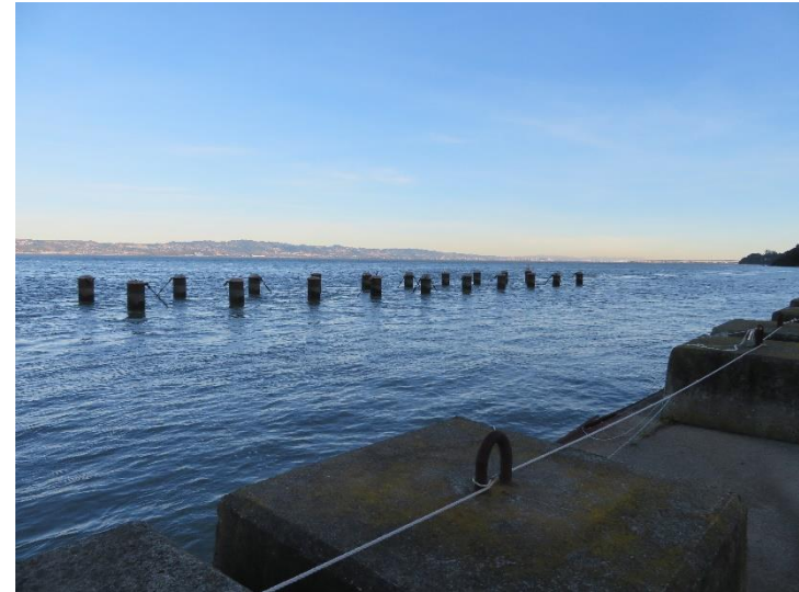
View of Caissons Offshore from Slab
