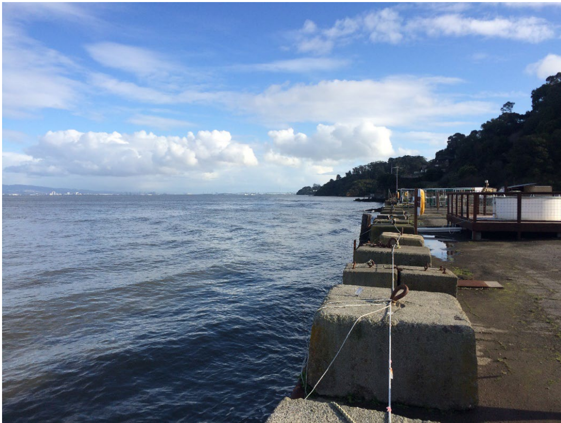
Figure 3. Quartered sea surface due to wave reflection off existing bulkhead (Source: ESA, 2019)
