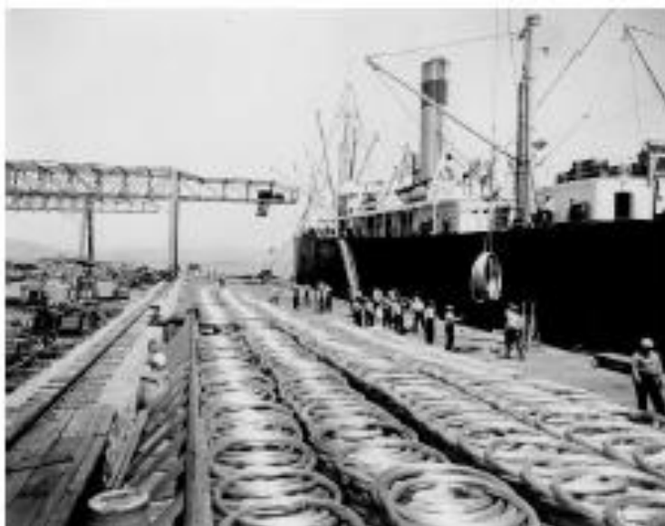
1933-1942 John Roebling's Sons Co - reeled suspension cables for Golden Gate Bridge
