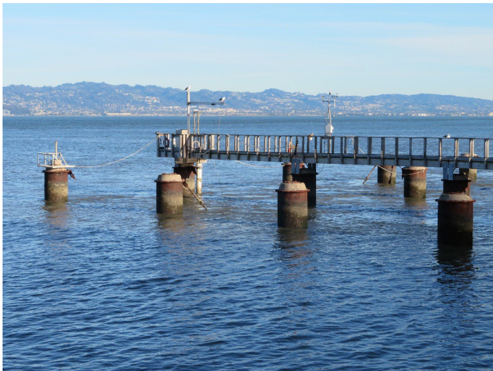
Figure 2. Existing research pier and caisson piles (Source: ESA, 2019)
