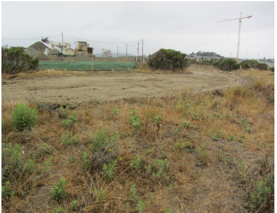
Top: Front end loader blading weeds outside the northern restoration area.
