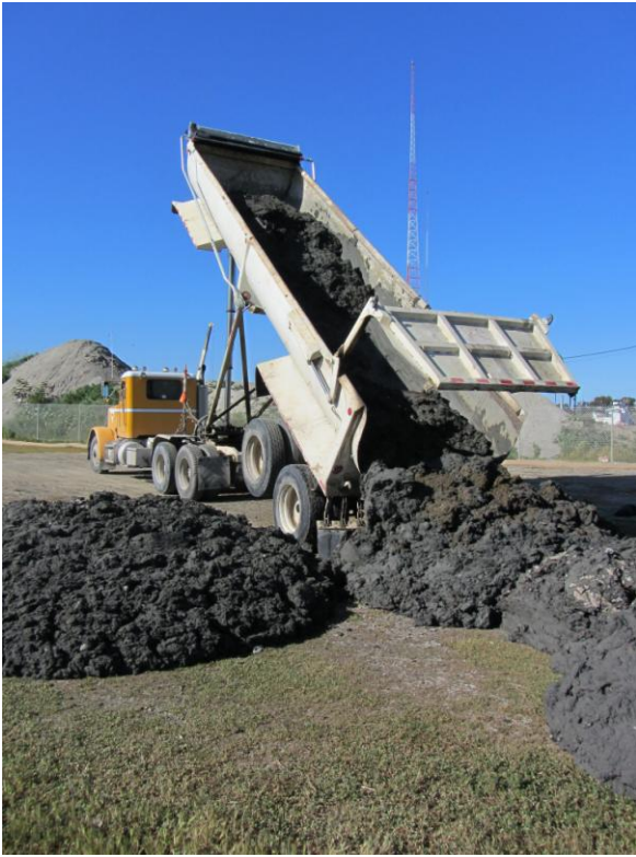
Above: Delivery of trucked in sediment.
