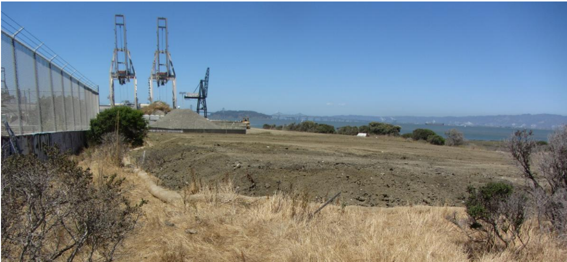
Top photo: Delivering sediment to the site. Bottom photo: Site after grading.
