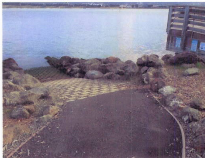
Figure 2. Steep Bank Access through Rock Cribbing
