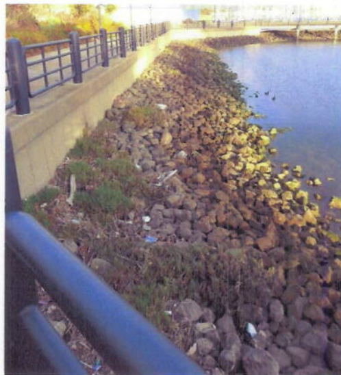
Figure 10. Boat Launch Pier Rip-Rap
