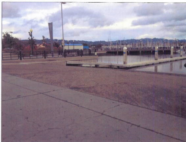
Figure 9. Boat Launch Pier
