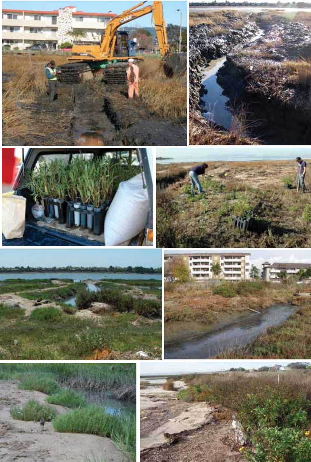
Figure 6. Channel construction and Grindelia planting at Elsie Roemer Wildlife Sanctuary, Alameda. Channels with berms were built in 2006 to provide marsh elevations suitable for native marsh vegetation after removal of extensive hybrid Spartina meadows. Grindelia was planted in 2007 and 2008, and annual and perennial pickleweed established naturally. In 2011, once the hybrid was predominantly under control, experimental plants of Spartina foliosa began (figures 4 and 5).
