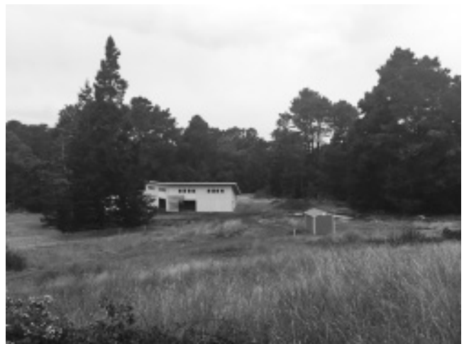
BUNKHOUSE VIEW FROM TRAIL.
