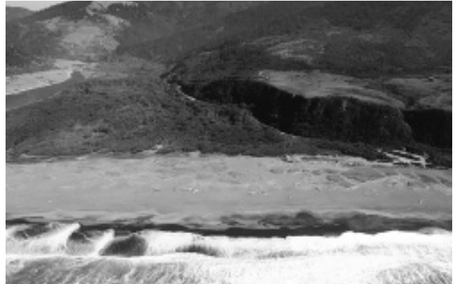
AERIAL VIEW OF PROJECT LOCATION.
