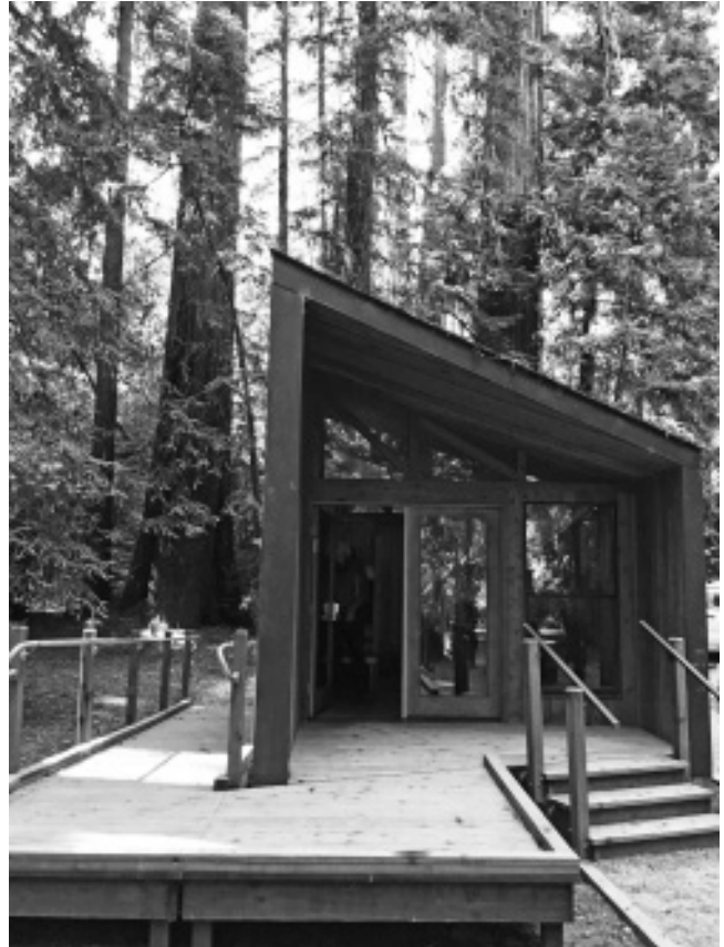
MODEL WEDGE CABIN AT PFEIFFER BIG SUR CAMPGROUND.
